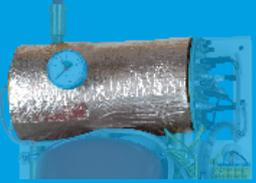
boiler insulation – mineral wool
